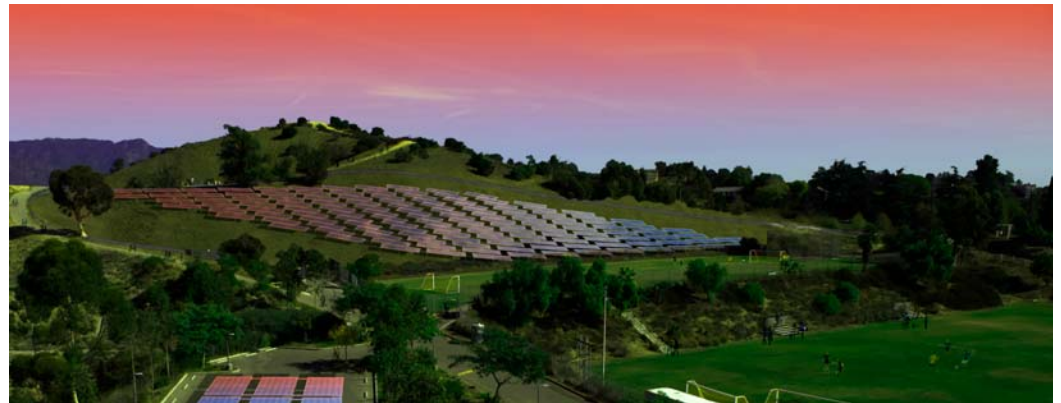
1MW Solar Array, Occidental College
