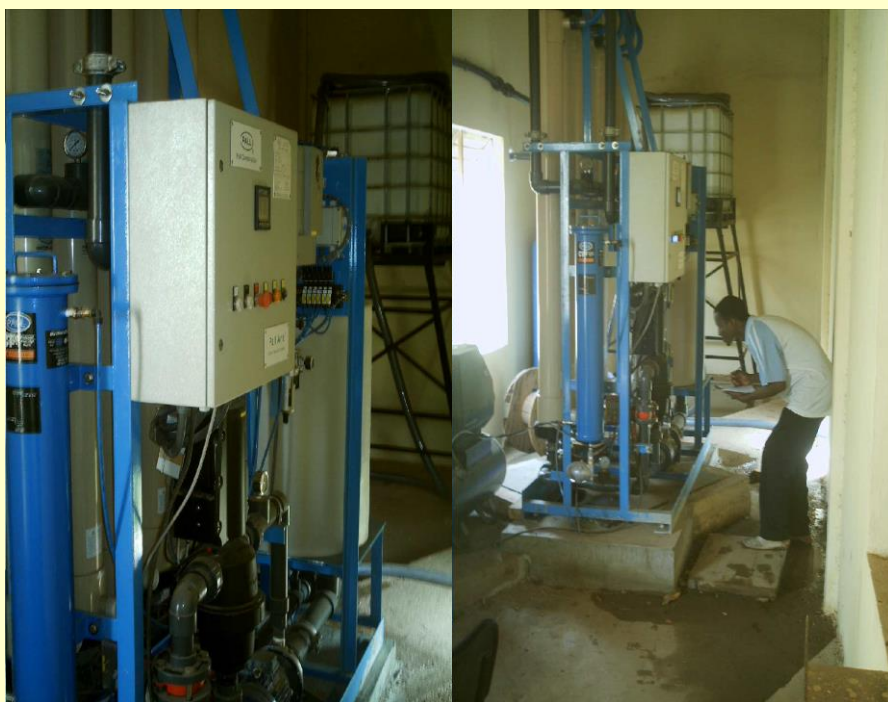
Pall Aria MF/UF unit AX2 Bamako, Mali
